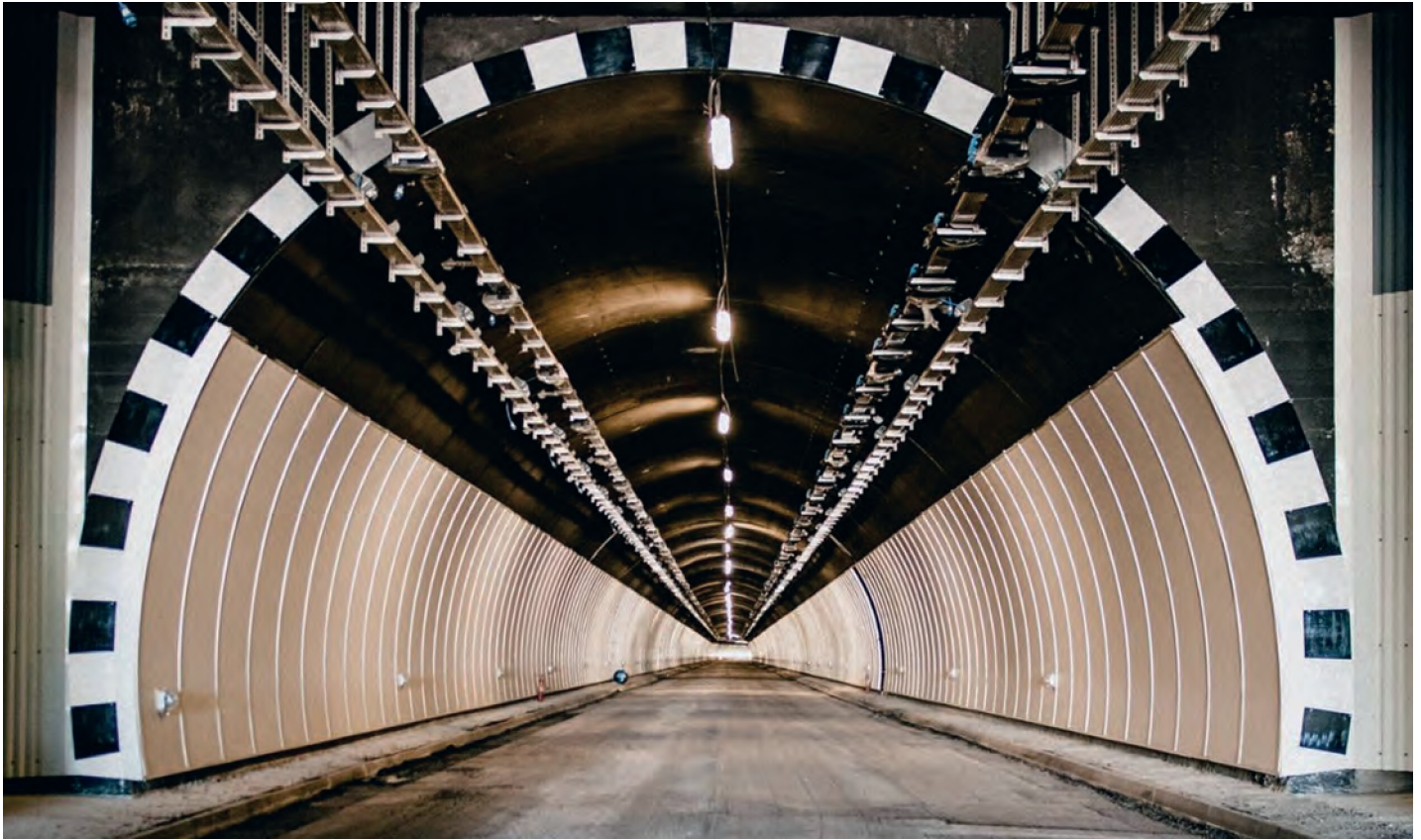
Newly completed tunnel in Gravina, Puglia.
